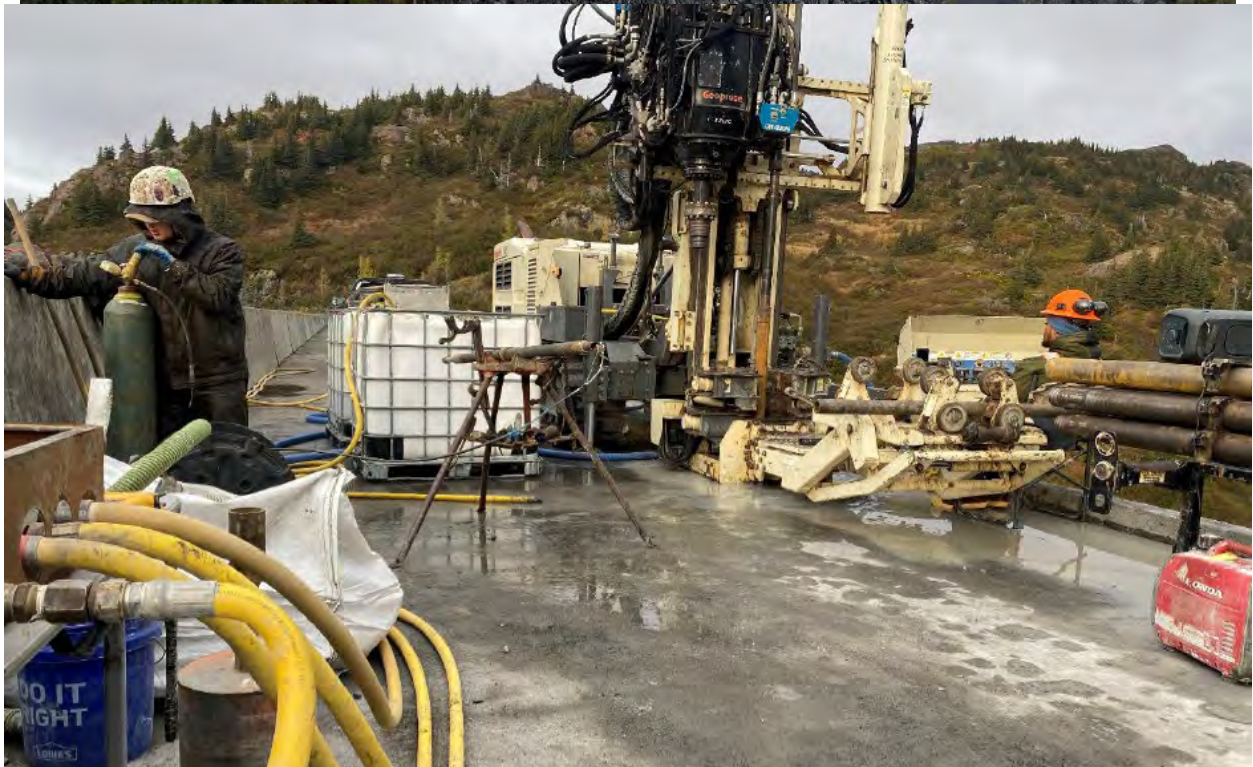
Drilling on Bradley Dam Crest
