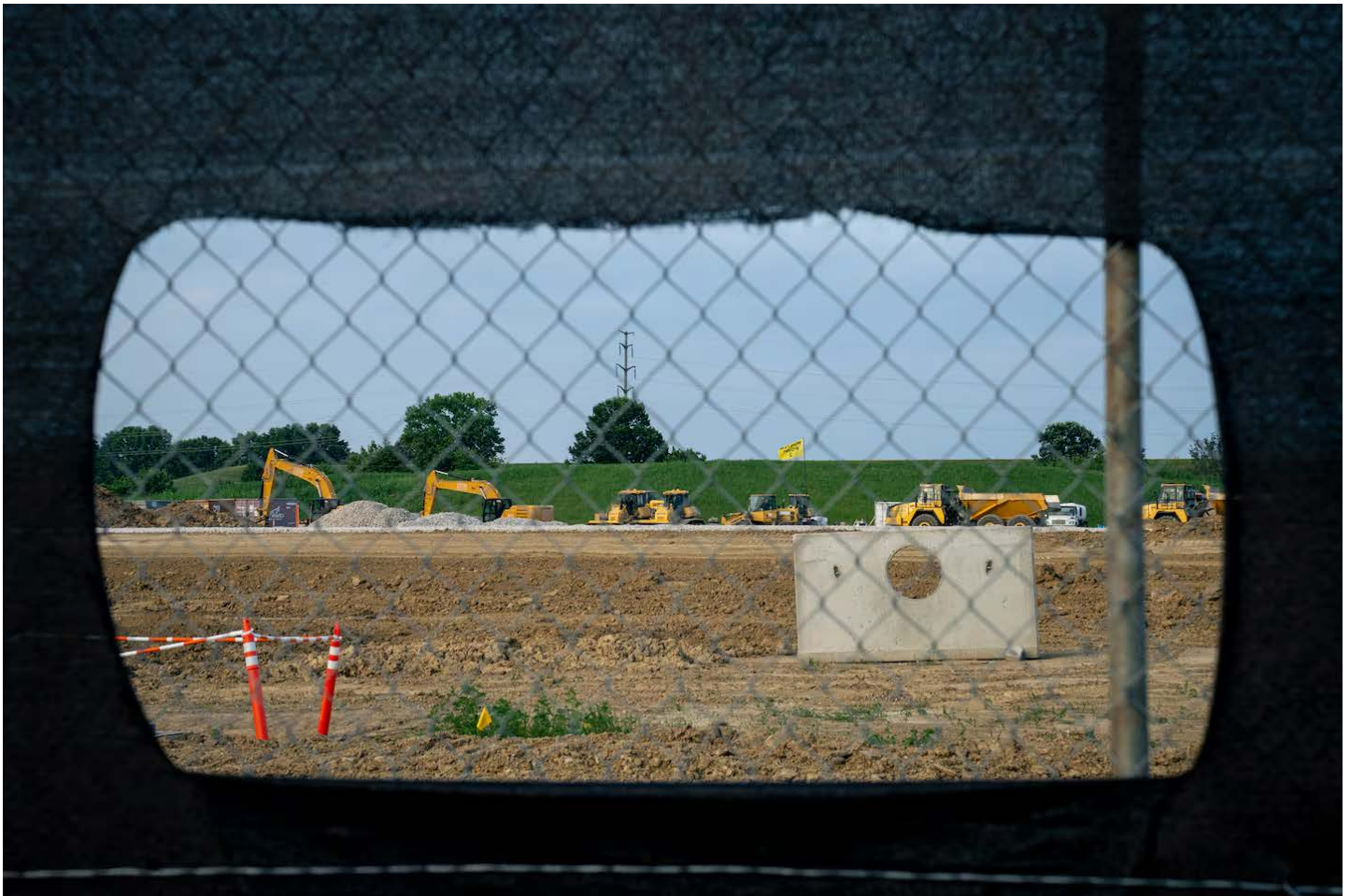
Construction equipment dots the landscape in Lewis Center, Ohio, where the COL5 will be a 480,000-square-foot data center. (Eli Hiller/For The Washington Post)
