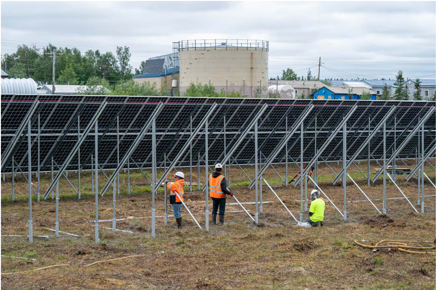
Workers with Alaska Native Renewable Industries construct a solar farm on in 2021 in Shungnak. The project includes 223kW of solar production and a 280kWH battery system. (Loren Holmes / ADN)
